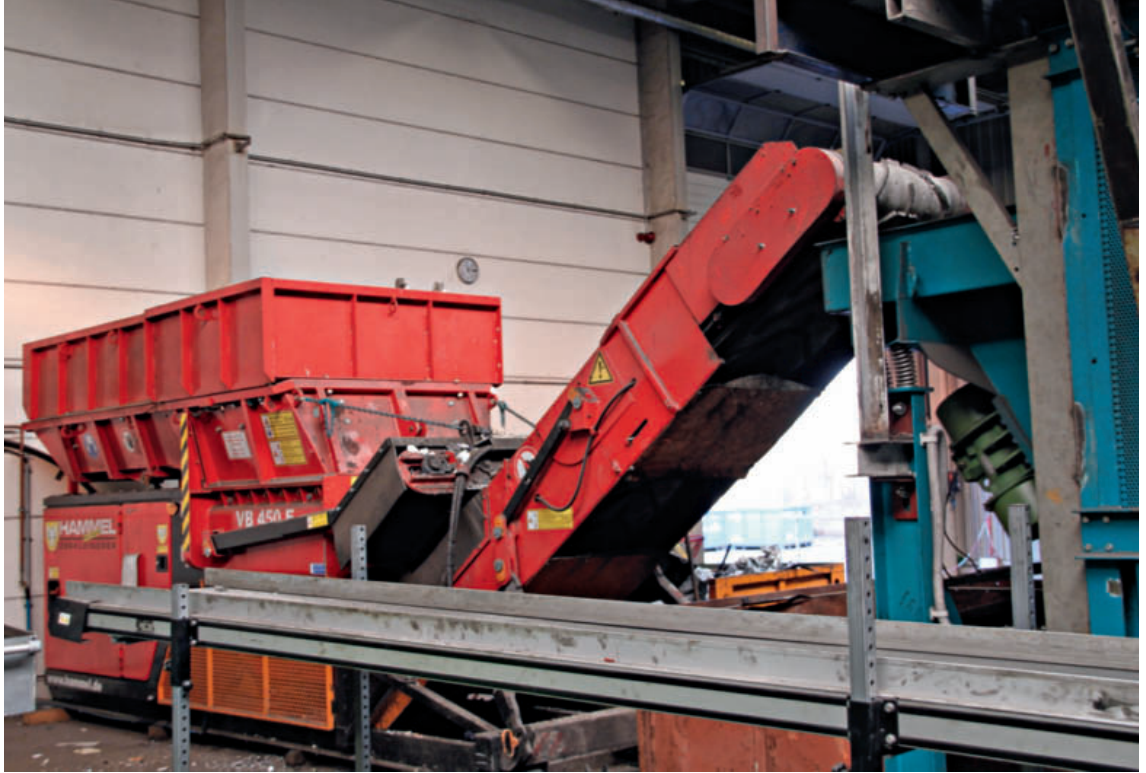
HAMMEL primary crusher VB450E with FE separation
