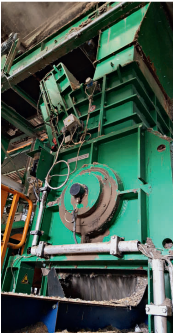
Used granulator before replacement
