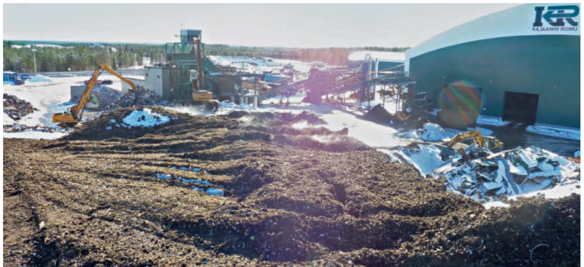
6 ▲ Loaded ASR input material with a particle size between 0 and 30 mm at the Kajaanin Romu Oy facility
