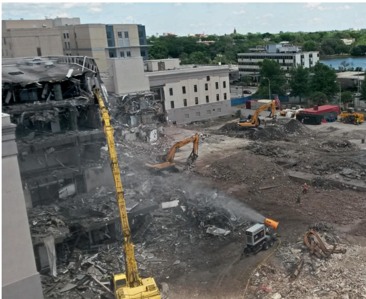
project), oversees the monitoring and compliance of fugitive dust emissions for the site. Jones used a hand held personal dust monitor to measure and record particulate emissions at 14 points, both on the ground and on rooftops of the surrounding facilities. He also regularly monitored air intake filters of surrounding MUSC facilities for signs of increases in particulate matter.
