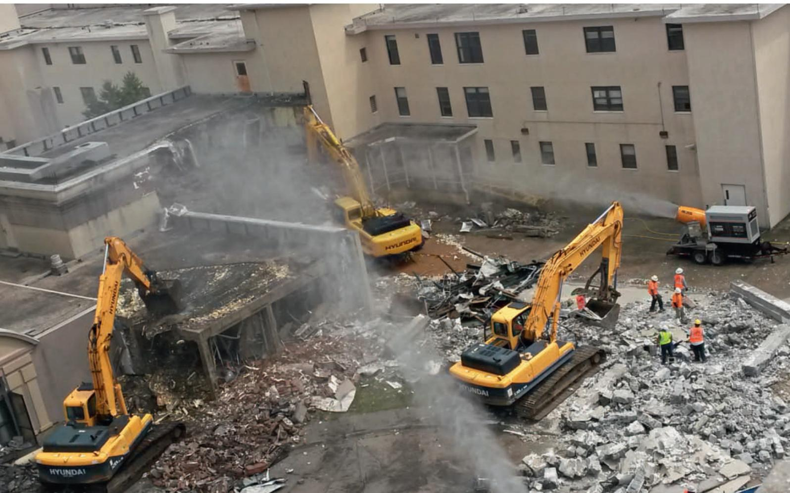
largely limited to surface suppression and the runoff can lead to wastewater compliance issues. Only atomized mist is capable of offering both airborne dust control and surface suppression over a large area, without saturating debris and causing extensive runoff.
