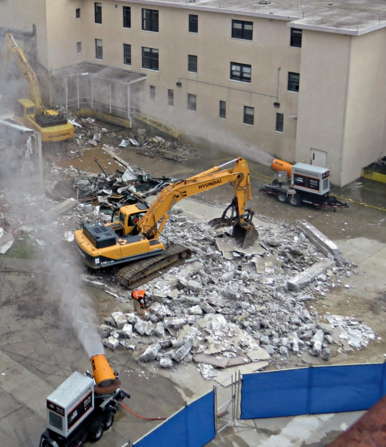
◀ Surrounded by buildings on all sides, the concrete buildings are carefully broken down by excavators
